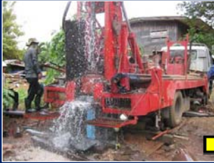
Drilling and Well Completion (Casing and Slotted placement)
