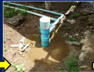
Completed well (waiting for well construction)
