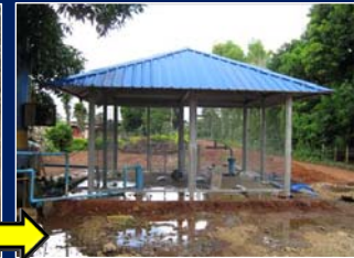
Building groundwater well
